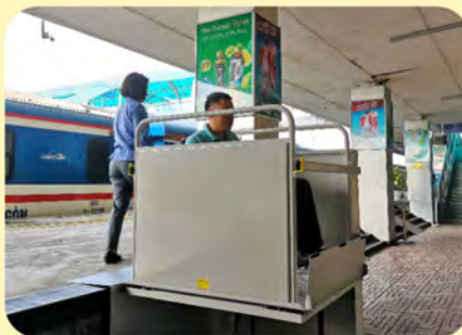
A station attendant tries out a "Wheelchair lift" installed at Hanoi Railway Station.
