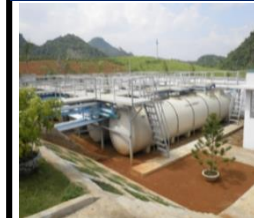
← Large Johkasou (250m 3 /day) installed in a public hospital in Vietnam.
