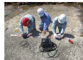
護岸の点検・補修
