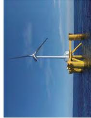
A 7-megawatt floating wind turbine has been constructed off the coast of Fukushima under a project commissioned by the Ministry of Economy, Trade and Industry. The blades reach a height of 200 meters (about 660 feet) above the ocean.
